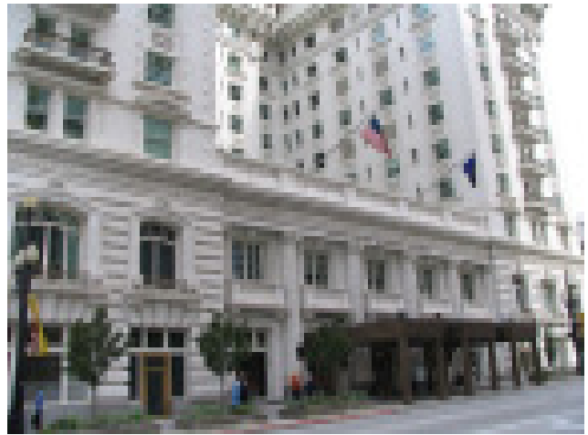
Church building that was formerly the Hotel Utah
